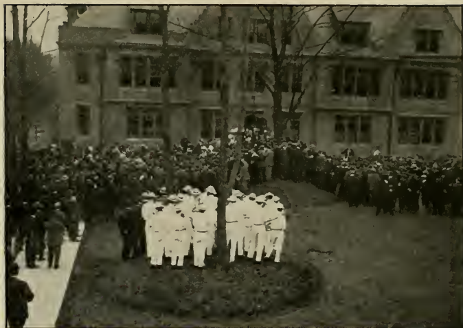
INSPECTING TAYLOR HALL
